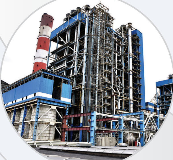
660 MW Super Critical Steam Generator – NTPC Solapur Thermal Power Plant
